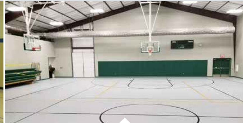
BLUM ISD Blum, TX Installed 2017
