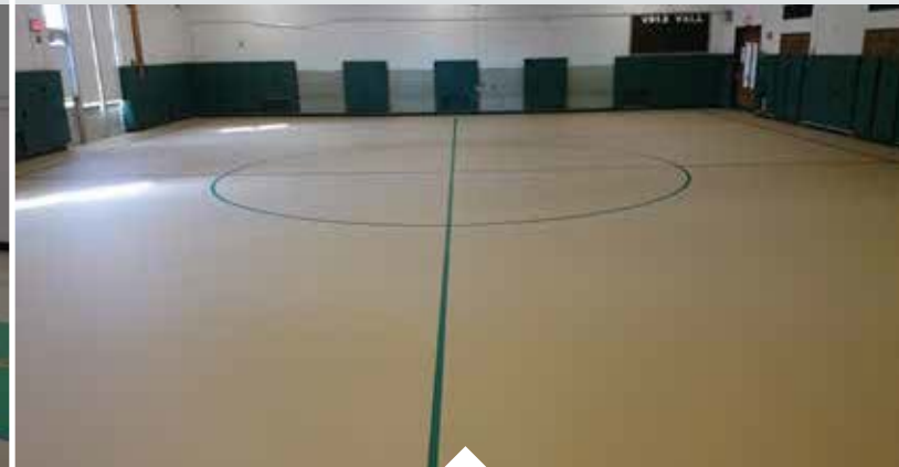
HILLSIDE ELEMENTARY SCHOOL Hastings-on-Hudson, NY Installed in 2016
